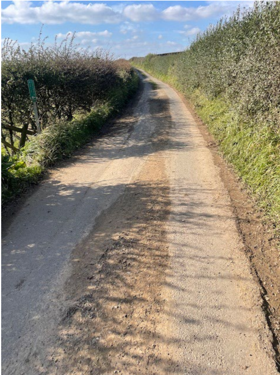
High Lane looking west
